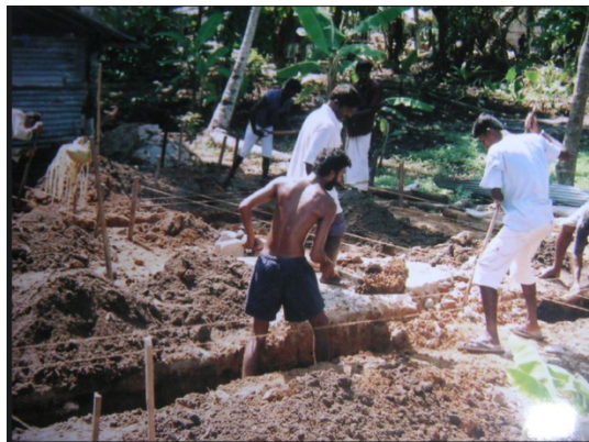
Photo credit: " Digging a foundation " by Sarvodaya Sri Lanka , CC BY 2.0 .
